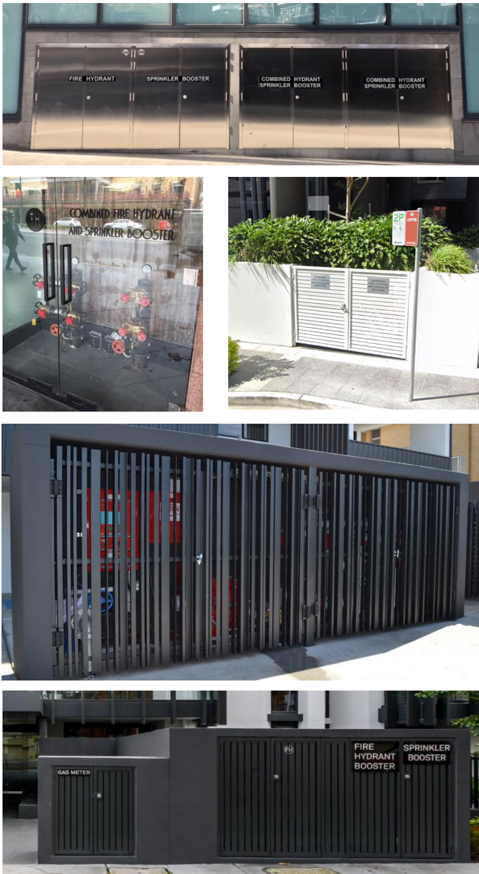
Figure 3. Examples of enclosed fire safety utilities
