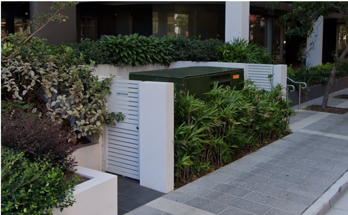
Figure 4. Example of a screened large power supply utility / substation
